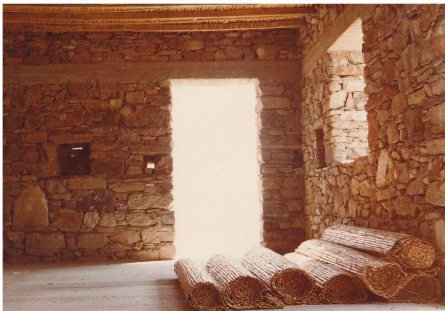
Villa T, under construction. Rolls of raffia used for the ceiling insulation, 1982. Courtesy Katerina Tsigarida Archive.
